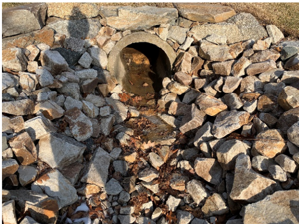
64 Gundalow - 1 (Drainage Course)
