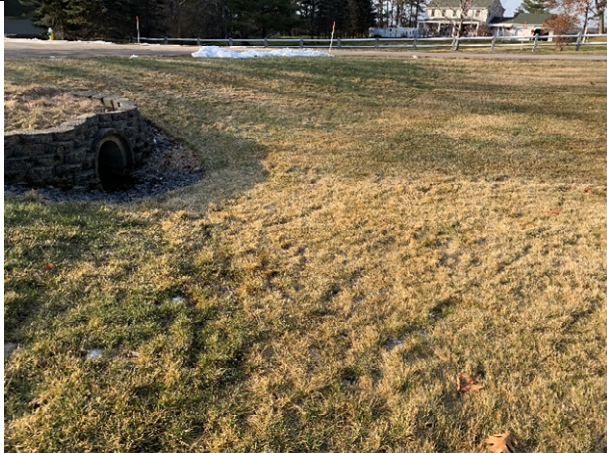
29 Gundalow - 1 (Drainage Area)
