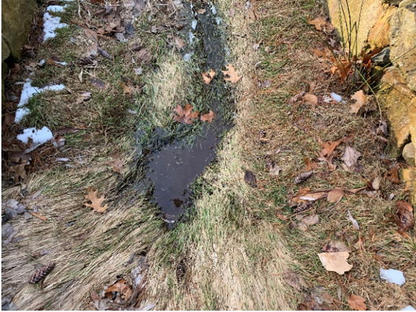
4 Brickyard Circle – 3 (Drainage Course)
