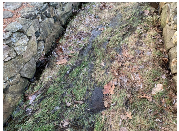
4 Brickyard Circle - 2 (Drainage Course)
