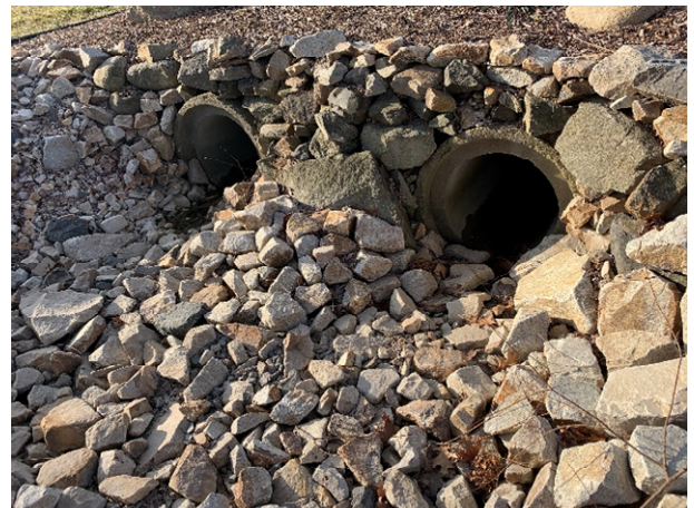
64 Gundalow - 2 (Drainage Course)
