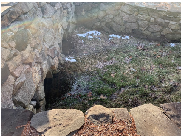
4 Brickyard Circle - 1 (Drainage Course)
